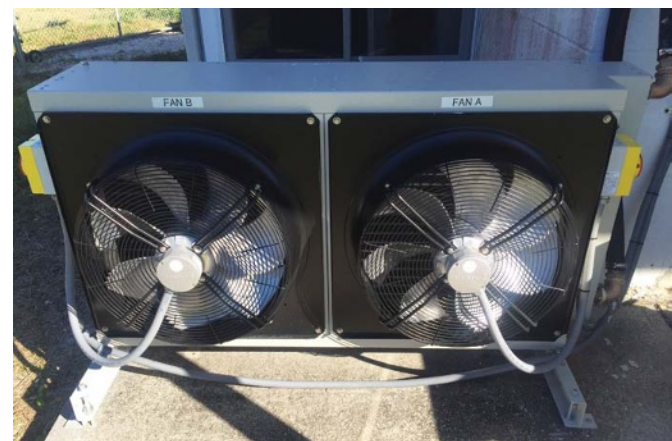
Fig. 1: The outdoor heat exchanger. A protective screen was added to the intake side to prevent dirt and grass from being ingested into its car-like radiator.
