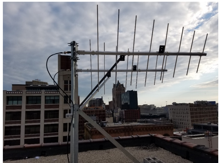
Figure# 3 Typical MaxxCasting or ZoneCasting antenna array (Shively 6025 dual)
